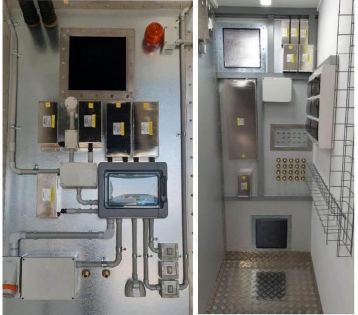
Single & three phase filtering, dedicated DC and signal line filtering.
