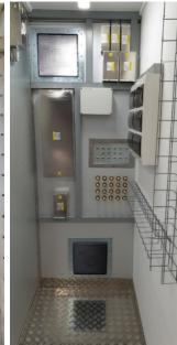
Single & three phase filtering, dedicated DC and signal line filtering.
